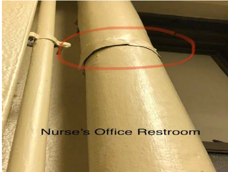
Not properly encapsulated
