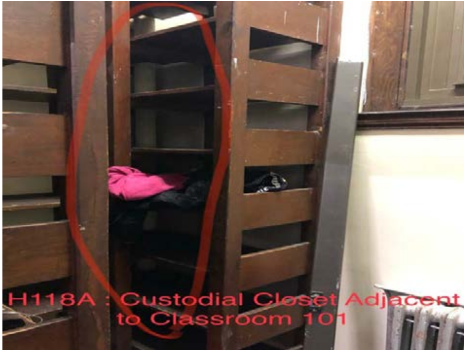
All pipe insulation needs to be abated
