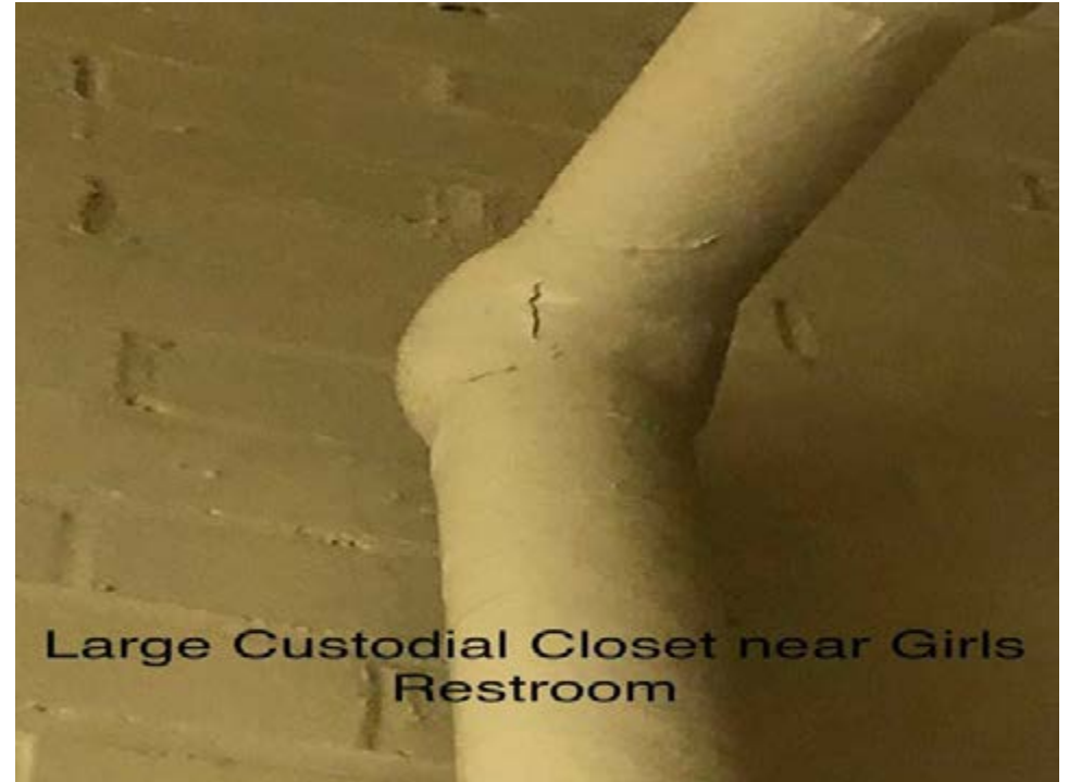
Cracked pipe fitting
