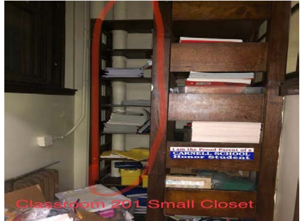
Remove all pipe insulation
