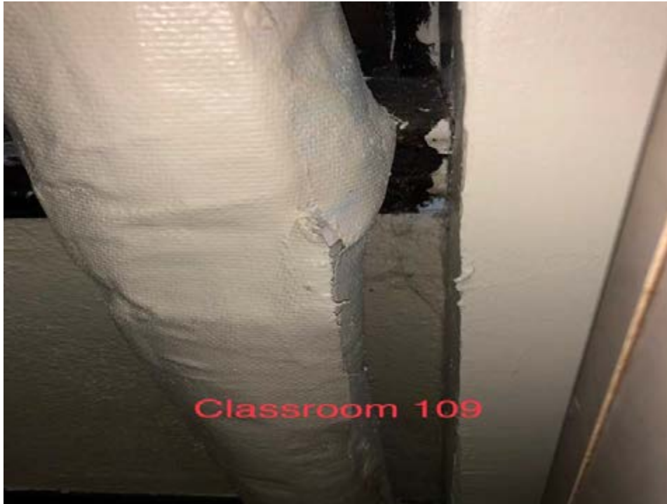
Wrapping becoming undone
