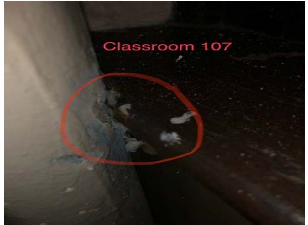
Small exposed section along window sill
