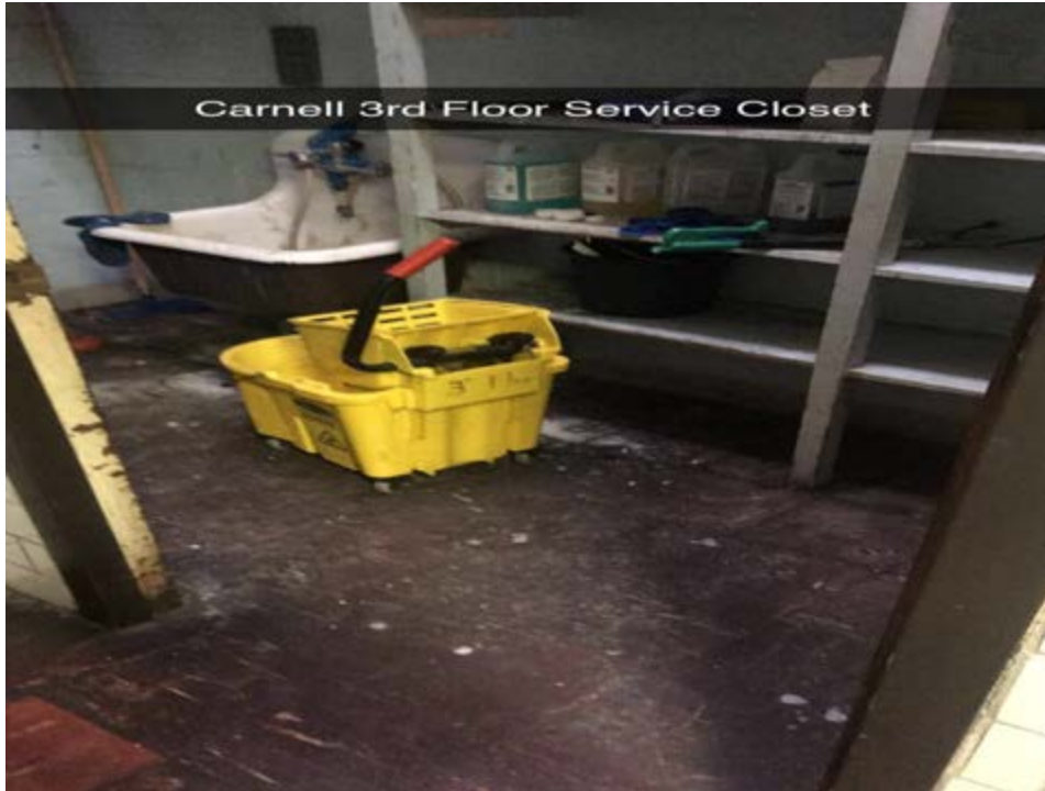
3rd Floor Custodial Closet
