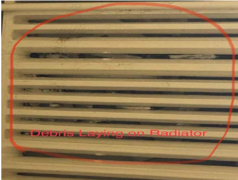
Debris laying on radiator
