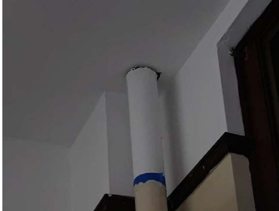
Exposed End At top of Riser
