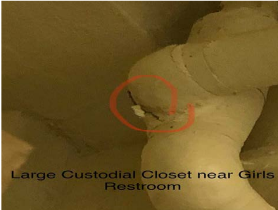
Cracked pipe fitting
