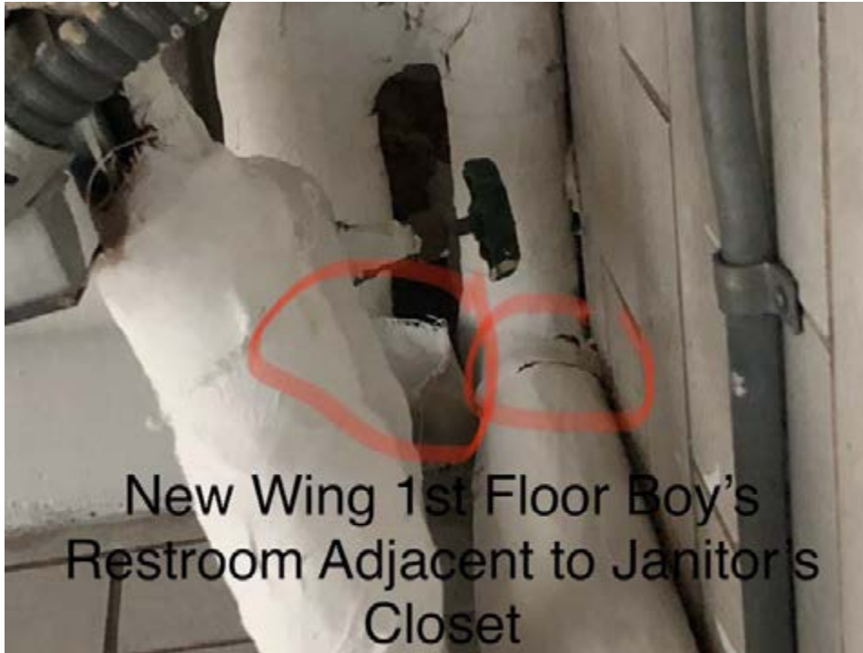
Crack in 2 Fittings
