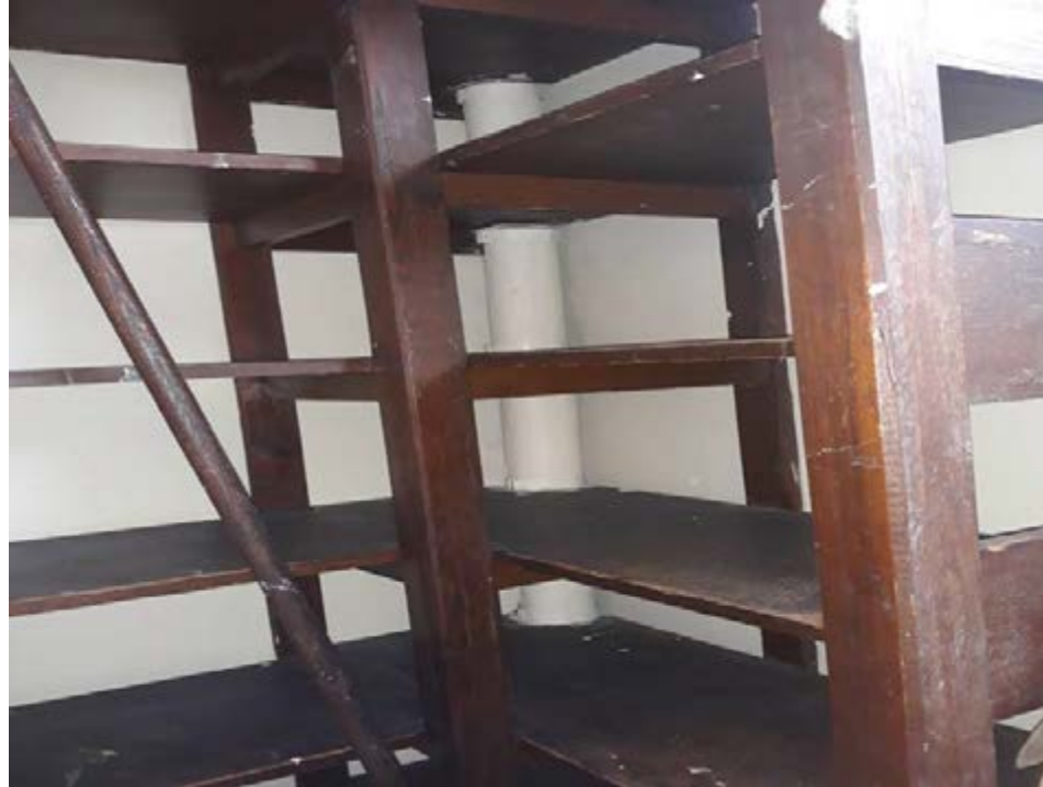
Bookcase Built Around Pipe Insulation
