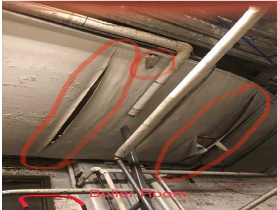
Tears in Seam and Insulation is sagging
