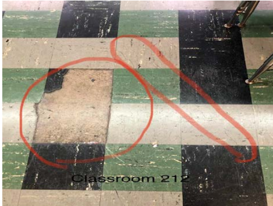
Cracks in tile
