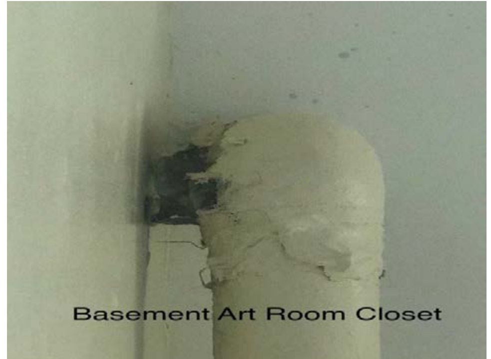
Significantly damaged fitting
