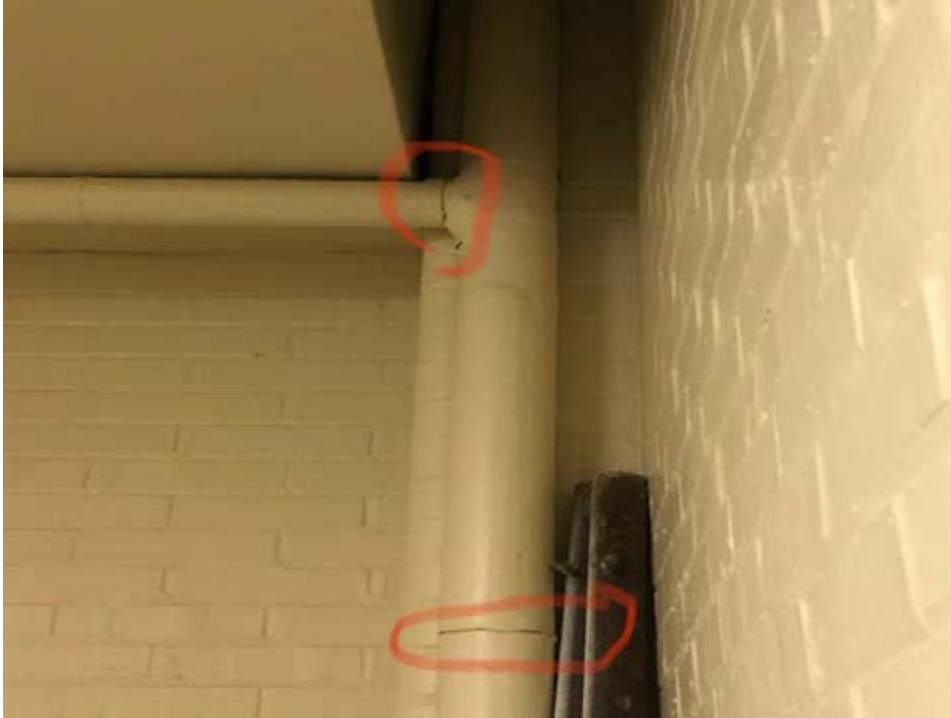
Two open seams in pipe insulation
