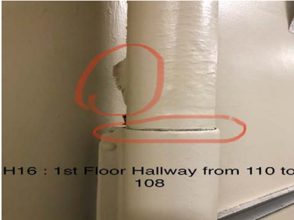
Seam opening and Wrapping becoming undone
