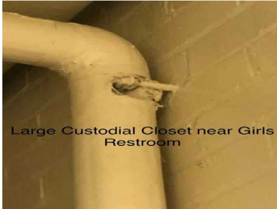
Exposed section of pipe insulation
