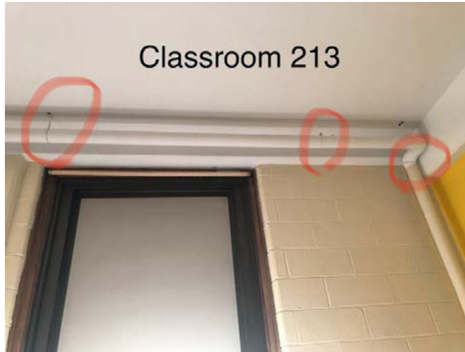
Perspective picture of cracked fitting
