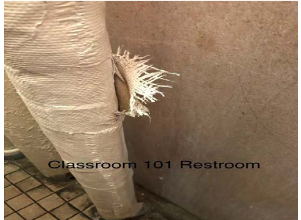
Wrapping becoming undone
