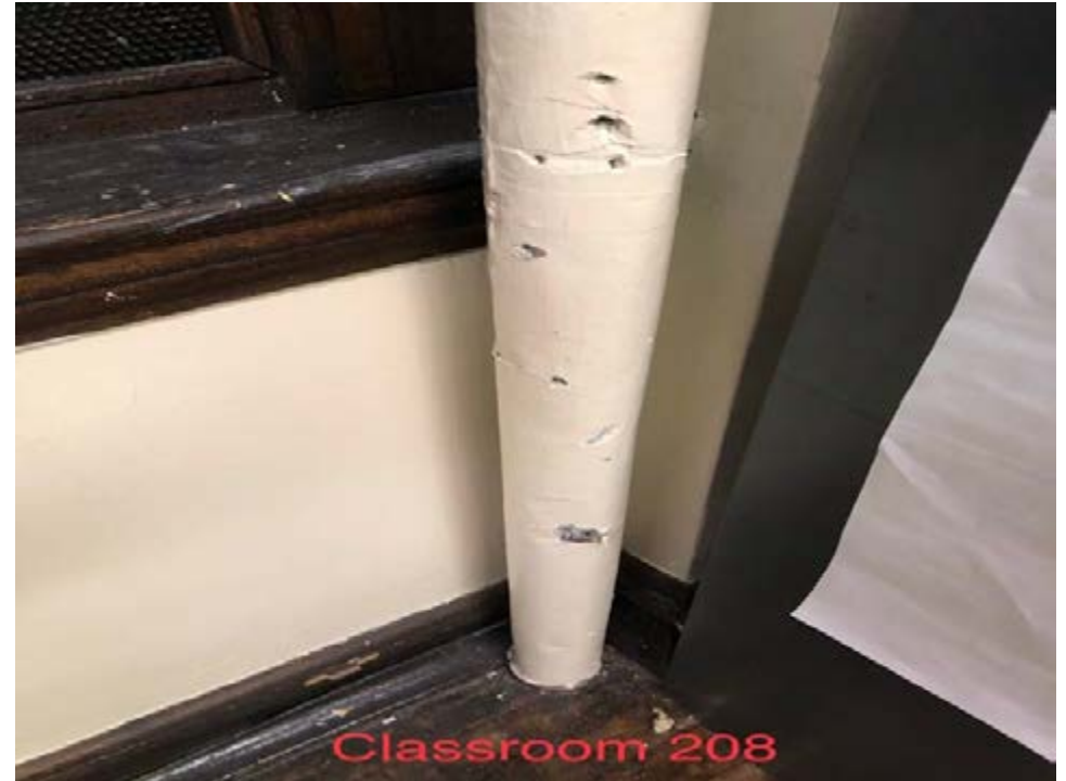
Picture of punctures and holes
