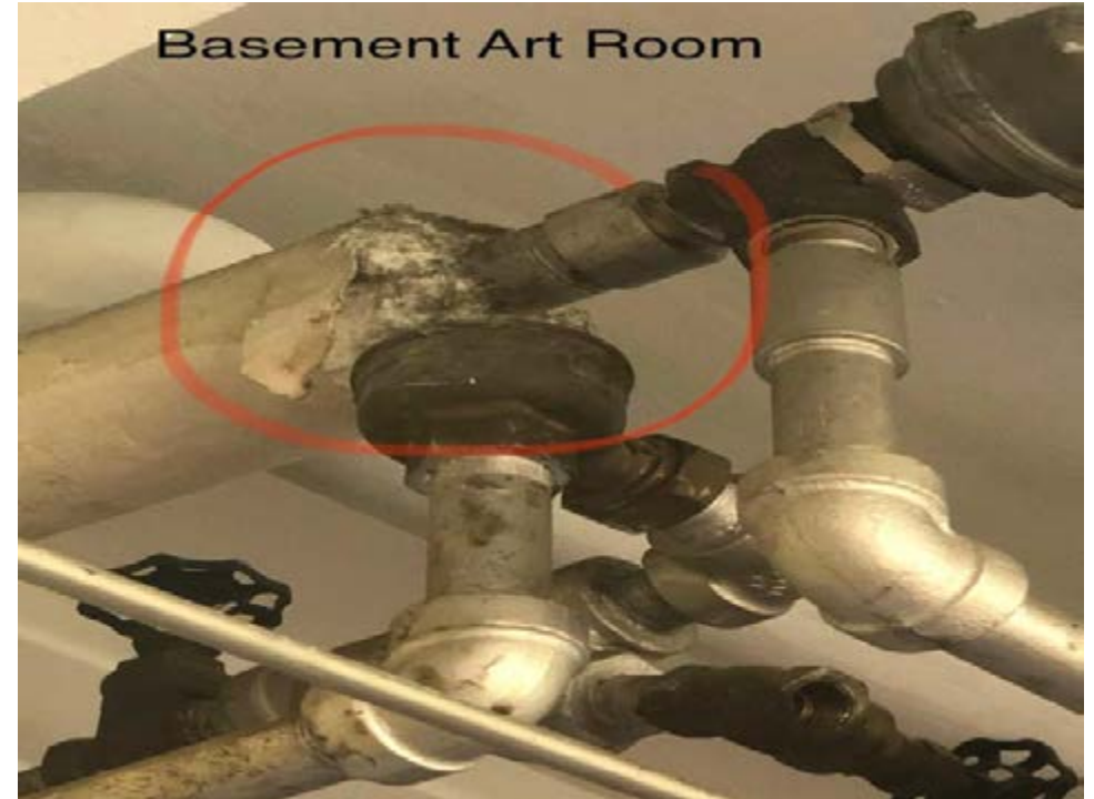
The Imminent hazard. Exposed asbestos mag insulation.
