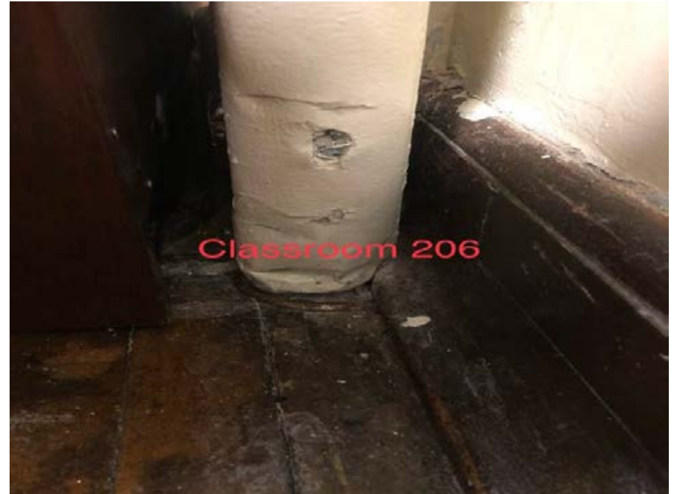
Punctured pipe insulation
