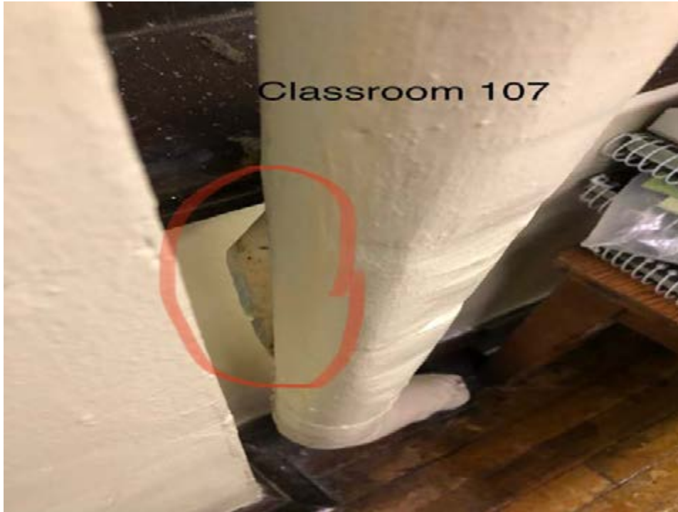
Wrapping become undone
