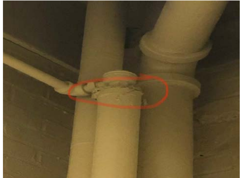
Exposed pipe end
