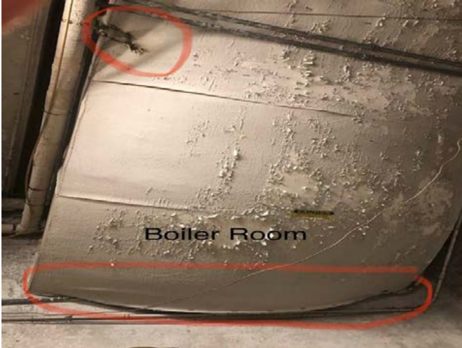
Tears in Seam and Insulation is sagging
