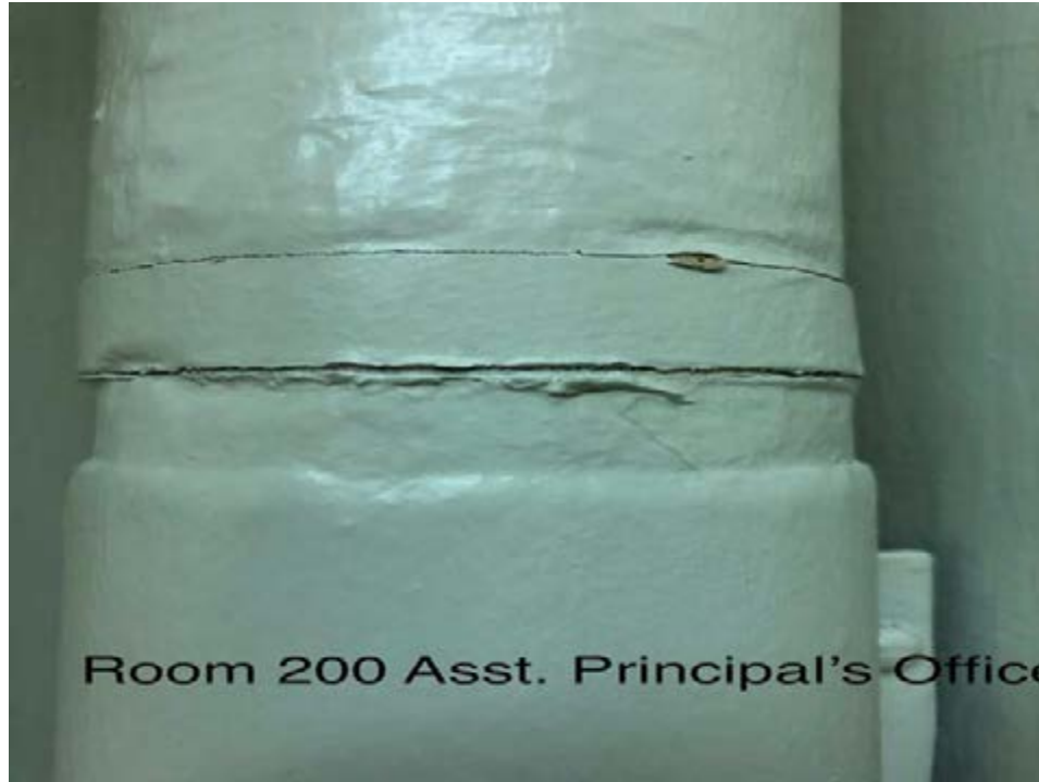
Open seam right riser
