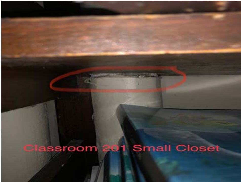
Damaged pipe insulation
