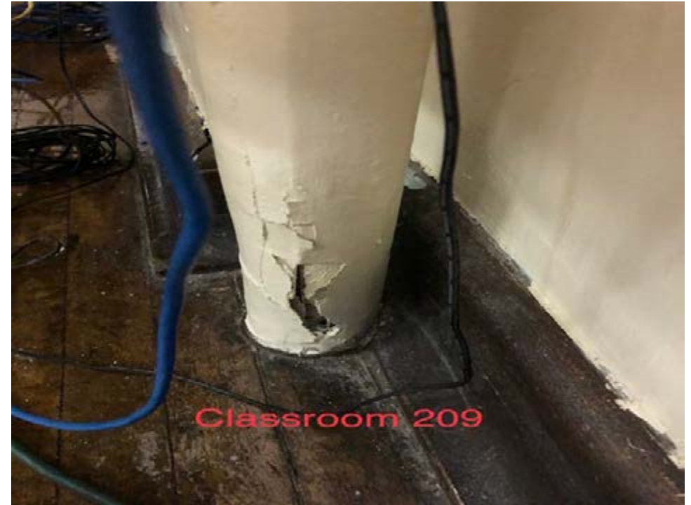
Large puncture exposing insulation
