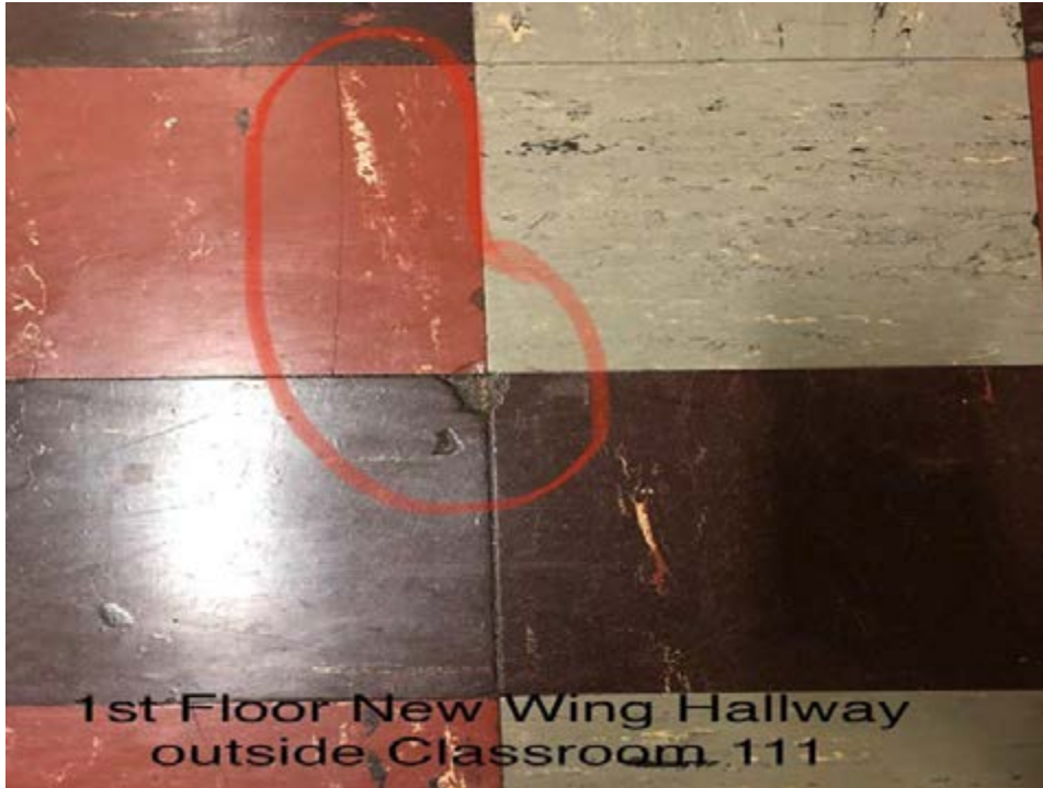
Cracks in Tile
