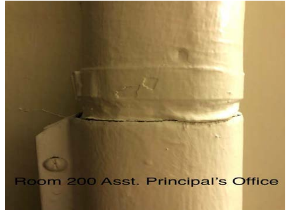
Open seam left riser
