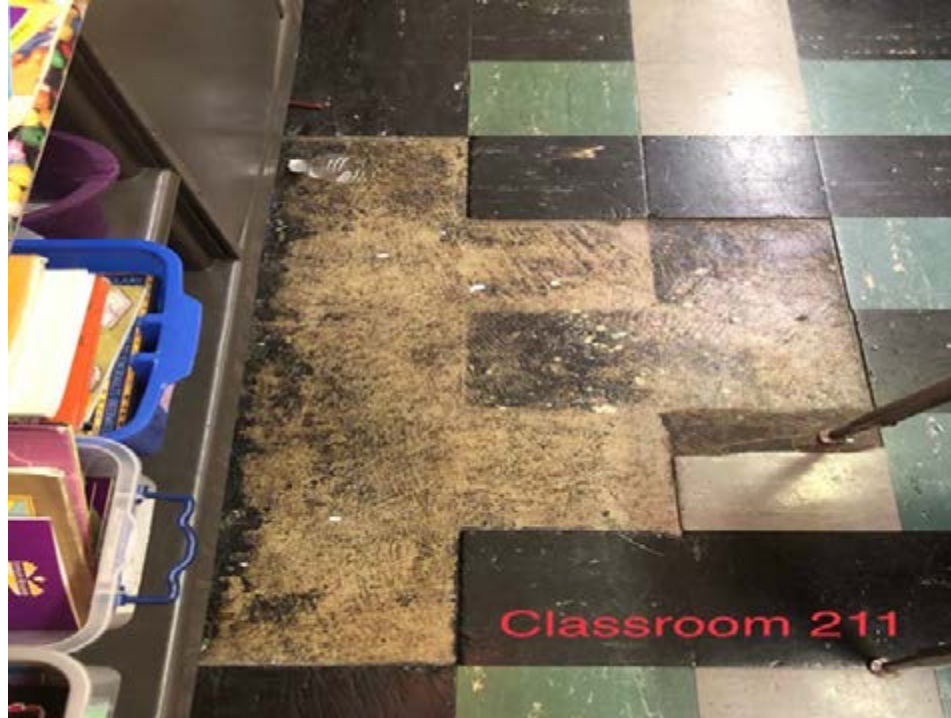
Cracked and missing tiles
