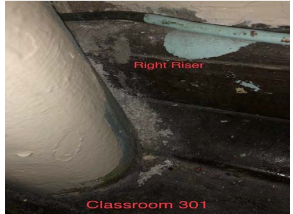
Debris around pipe and on the floor
