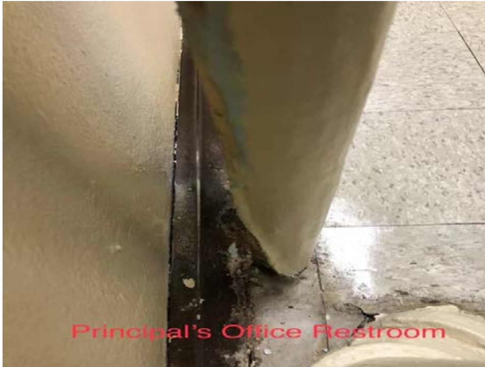
Wrapping becoming undone
