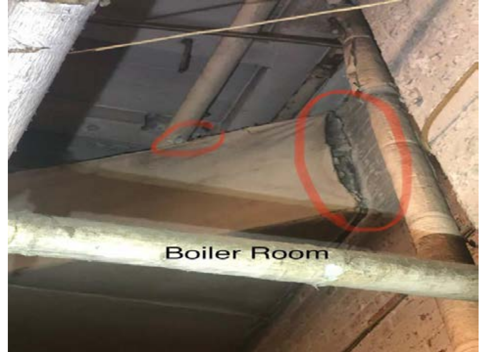
Tears in Seam and Insulation is sagging
