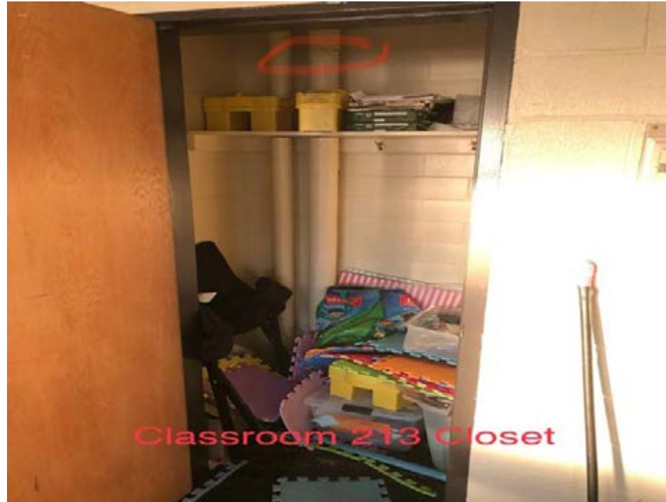
Perspective picture with open seam damage
