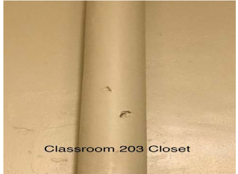
Close up picture of holes
