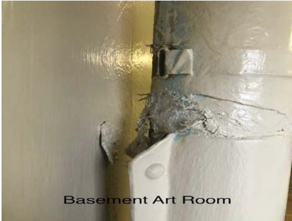
Exposed asbestos mag insulation
