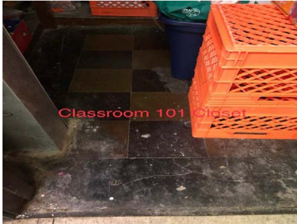
Cracking Floor Tile
