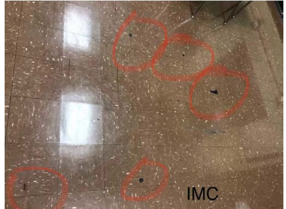
Cracks, dents and missing floor tiles
