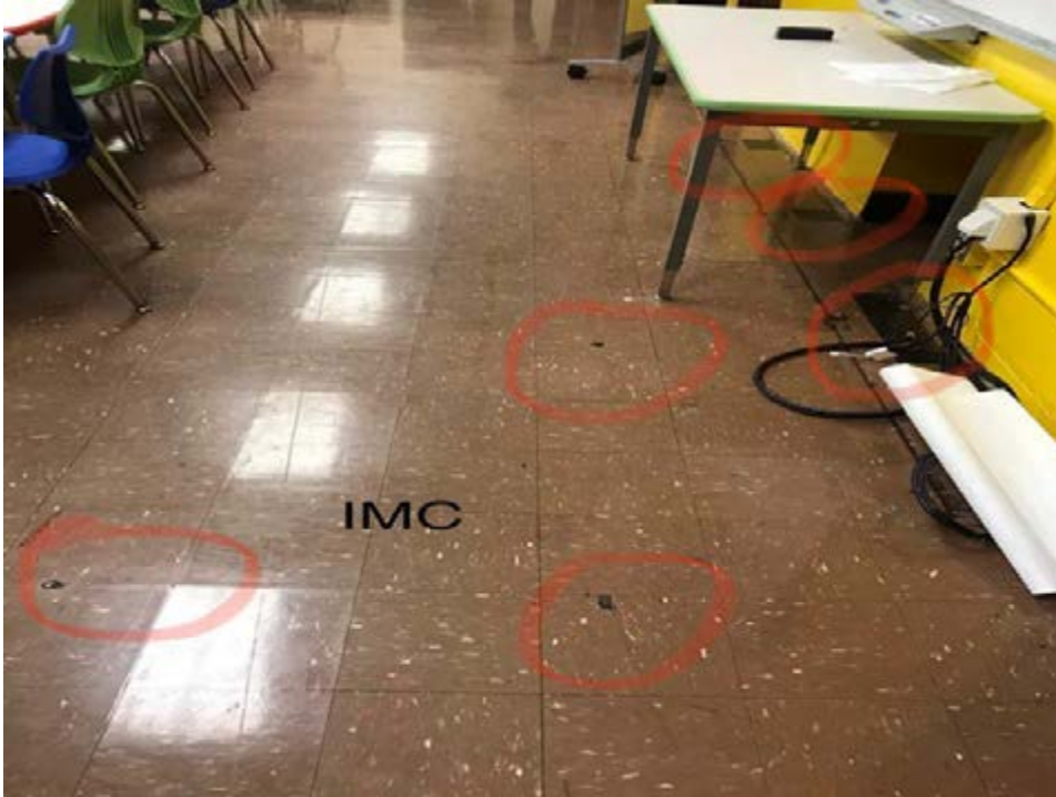
Cracks, dents and missing floor tiles
