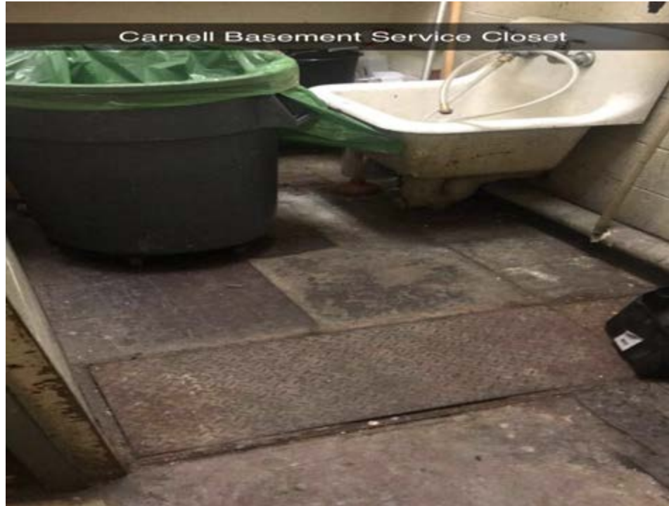
Custodial Closet in the Basement
