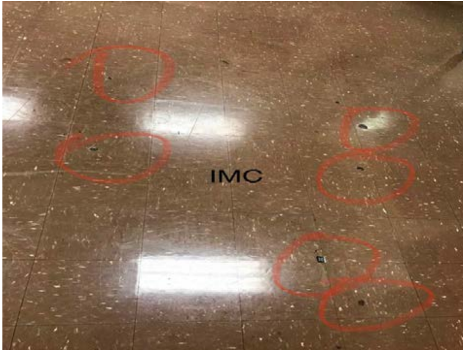
Cracks, dents and missing floor tiles
