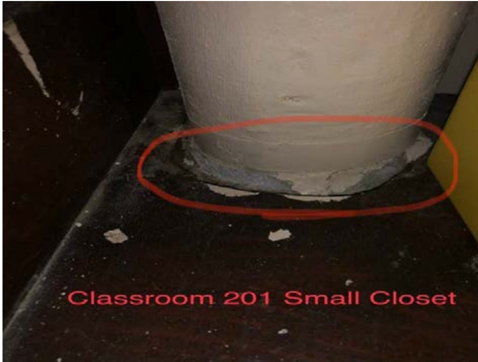
Damaged pipe insulation
