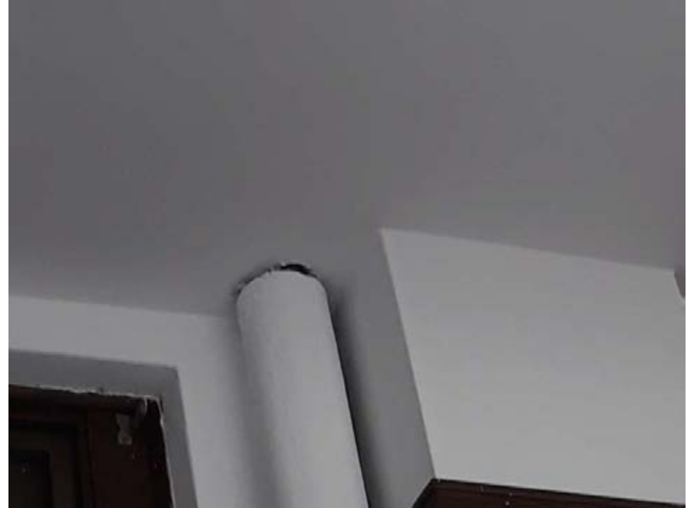
Exposed End At top of Riser
