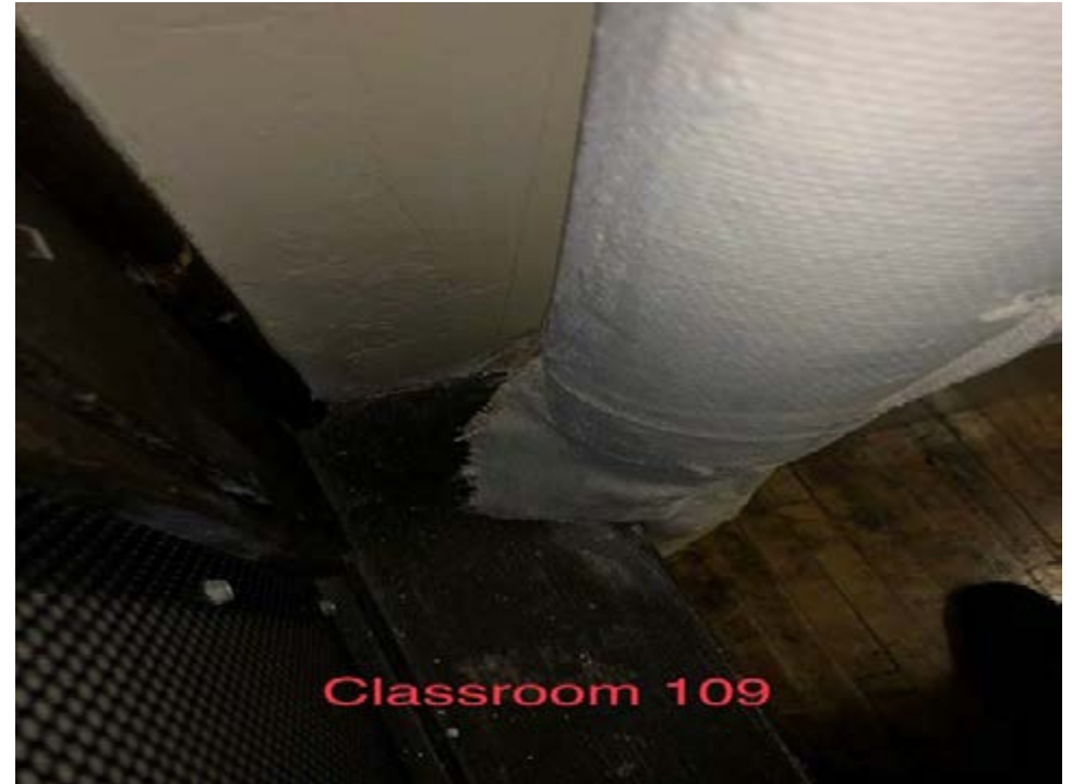
Wrapping becoming undone
