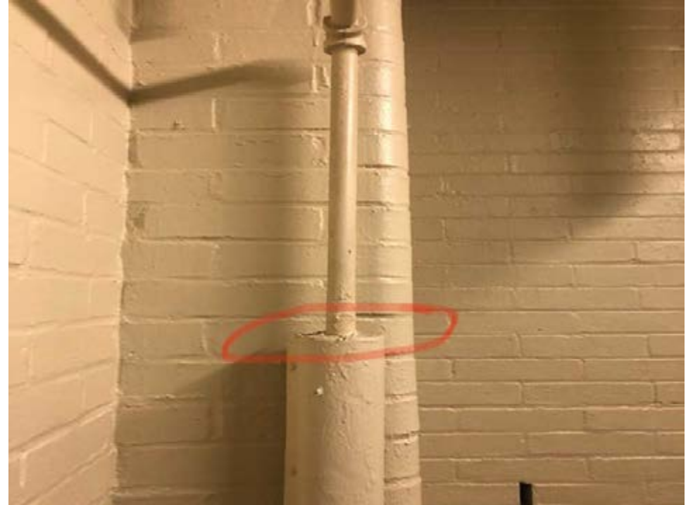
Open pipe end
