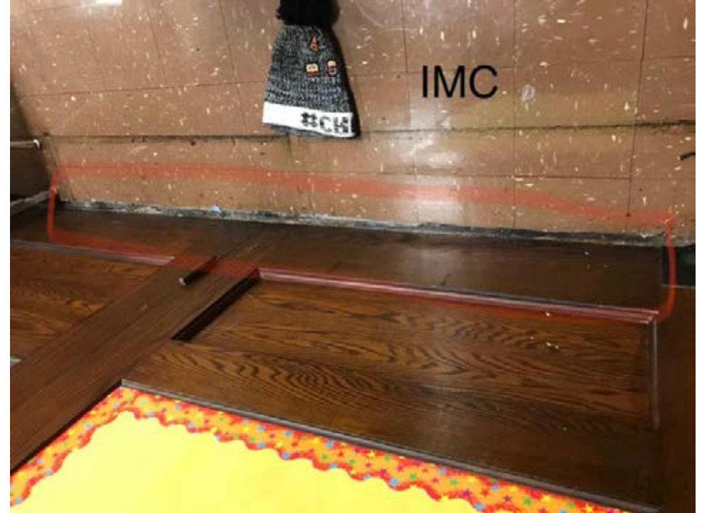
Cracks, dents and missing floor tiles
