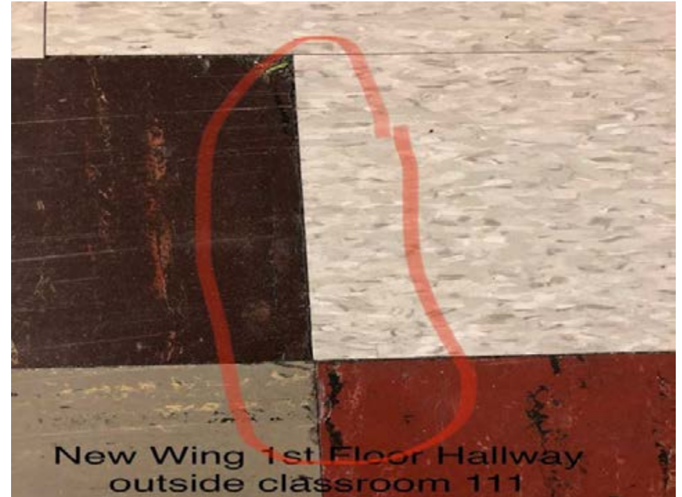
Cracks in Tile
