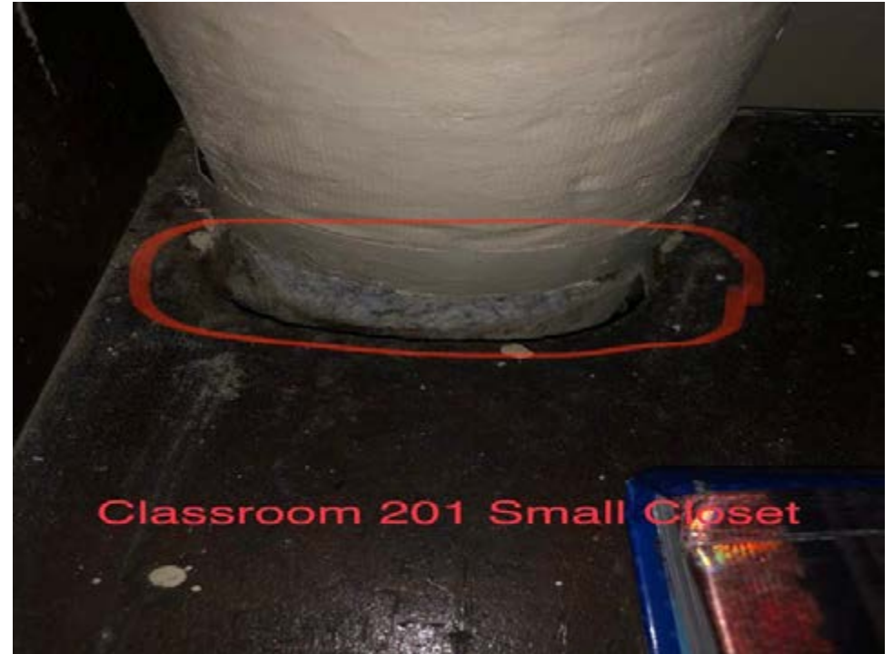
Damaged pipe insulation
