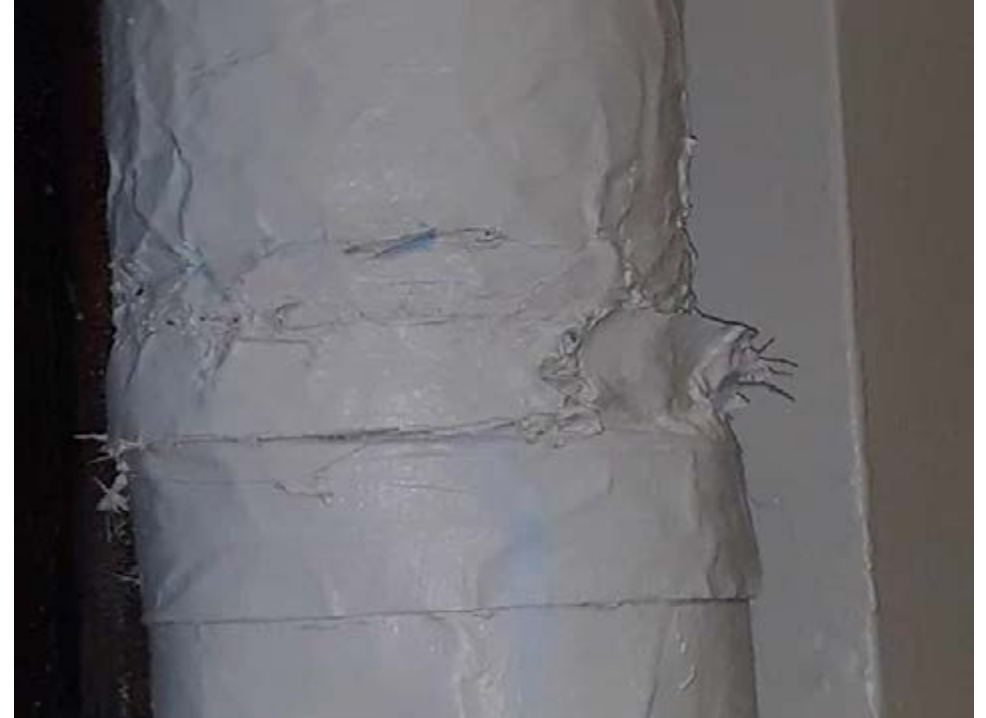
Crack in seam
