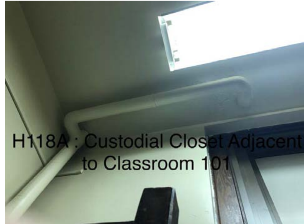
All pipe insulation needs to be abated
